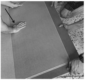
If difficulty to fit panels between each other, check that "fold/down" click system is not damaged or blocked.
