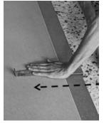
Place the pull bar support against the edge of the lower board so as not to damage the connection system.
