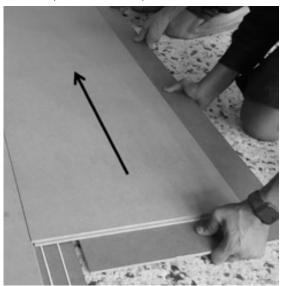
5. Clamp the length of the panel to the previous row using the pull bar and the mallet. The panels must be edge-to-edge.
