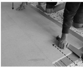
Place the pull bar support against the edge of the lower board so as not to damage the connection system. For a perfect panels fitting, it be may helpful to apply a load located near to the junction of the 2 panels previously installed.
